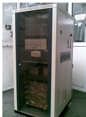
Product 3 - 5 kW integrated energetic system, based on fuel cells
